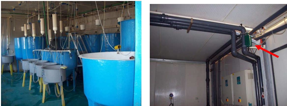
Figure 8: In these tanks (Right), new-born fish are placed to begin their growth. The Agriflow unit (right) protects the fish against bacteria, and also protects the heat exchanger against limescale.
